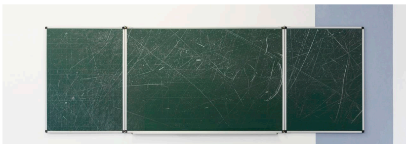
Before applying board film on board
